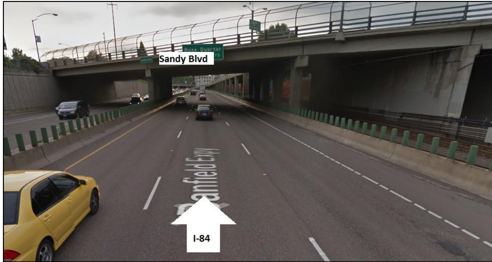
Figure 11: Sandy Blvd. Overpass at I-84 – Source (Google Maps)
