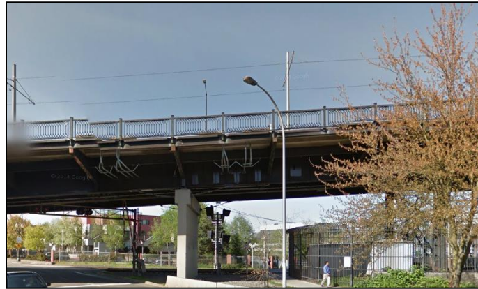
Figure 8: Utilities Under and Near the Steel Bridge – Source (Google Maps)
