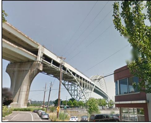
Figure 14: Fremont Bridge (I-405) with Nearby Power Lines – South End Source - (Google Maps)
